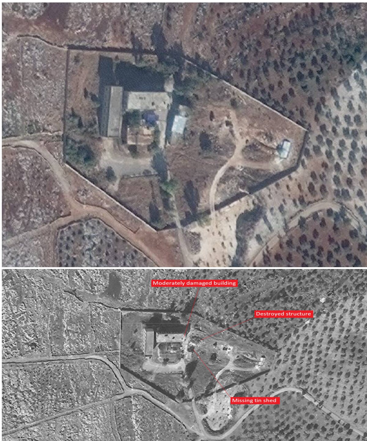
Top: Satellite image of the Al-Arashani water station, 12 November 2021©2021 Maxar Technologies.
