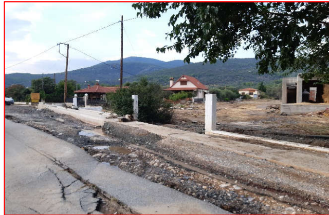
Collapsed and eroded road embankments, scoured asphalt deck.
