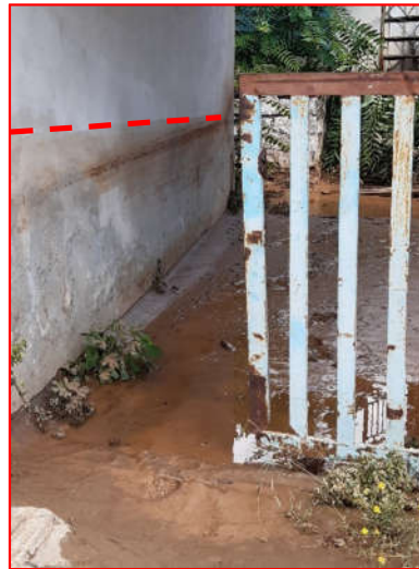
Water stage recorded at multiple locations around Psachna at 0,60m to 1,8m.
