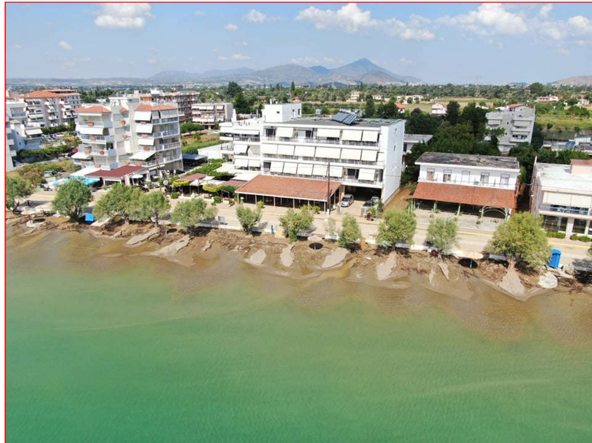
Erosion rills at Lefkanti beach
