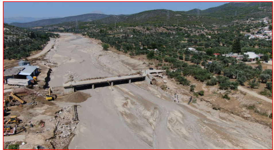
UAV images of Afrati Bridge
