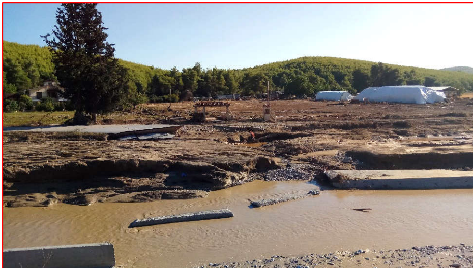
COLLAPSE OF BRIDGE BETWEEN POURNOS AND MISTROS
